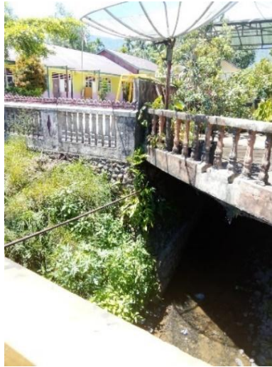
Figure 3. River in the vicinity of State Kindergarten 01 Koto Parik Gadang Diateh used as a toilet due to limited sanitation facilities
